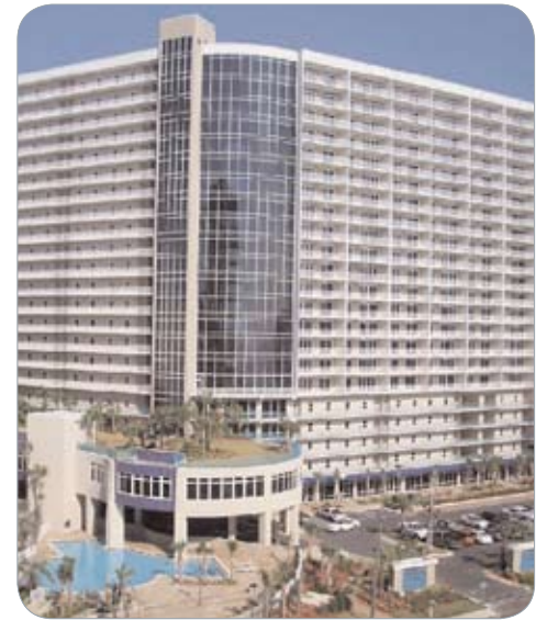
Construction and development of Laketown Wharf, the largest single-building condominium resort in Panama City, Florida, was completed this year after foreclosure in 2008.
